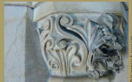
Cleaning general soiling from limestone using a latex poultice
