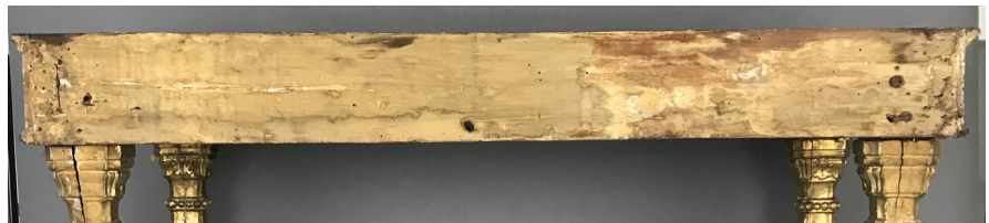
Fig. 24. Dovetail joinery in the exterior timber.
