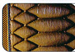
Ladies Withdrawing room wall by the door before conservation
