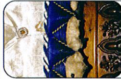
Day Saloon area above the door before conservation
