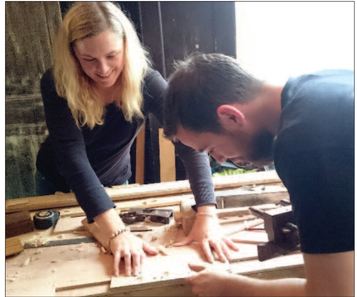
Timber panel repairs at Barnstaple with conservation carpenter and Fellow Ben Hornberger
