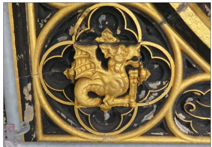
The Welsh Dragon on the North Clock Face before restoration began showing the 1983 decorative scheme
