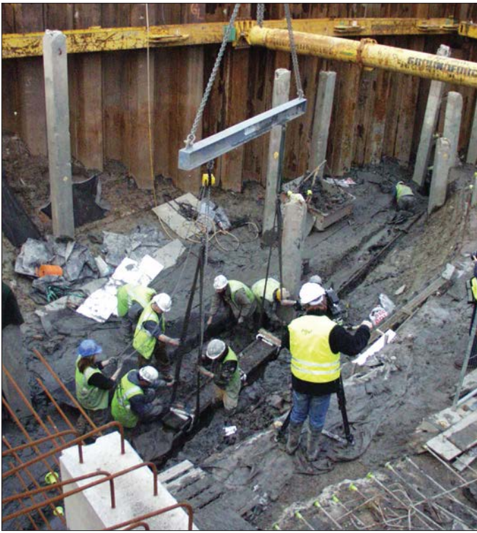
Archaeologists lifting a section of the keel. Between 5 and 7m of alluvial overburden had to be removed to fully uncover the ship before it was dismantled and raised
