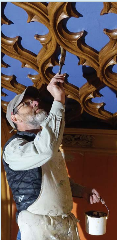
Graining the reticulated ceiling at St Mary's, Long Crichel, Dorset
