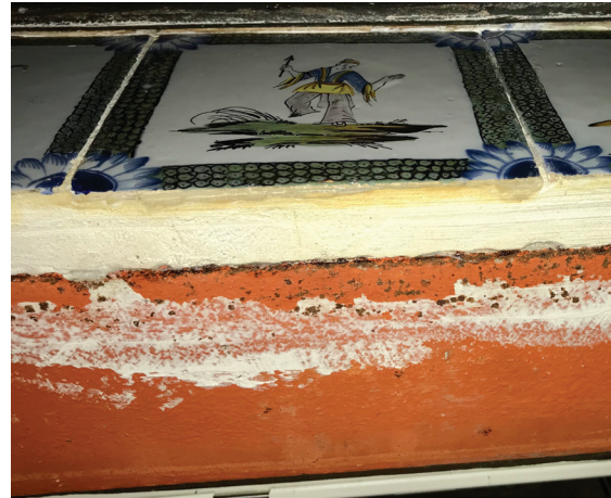
Figure 3. Bertrand Fireplace (left) and detail of plaster and steel armature (right), Winterthur Museum, 1969.4720.002 - 1969.4720.026 (clockwise from lower proper right) · Courtesy of Winterthur Museum, Garden & Library
