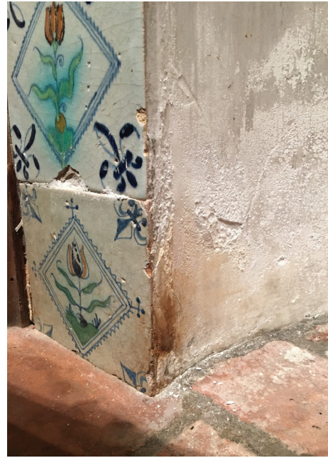
Figure 2. Vauxhall Fireplace (left) and detail of salt damage on the tiles and plaster surrounds (right), Winterthur Museum, 1969.4722.002 - 1969.4722.036 (clockwise from the lower proper right) · Courtesy of Winterthur Museum, Garden & Library
